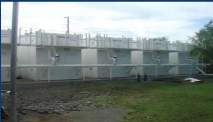
Installation of Transtank at Seaoil Malalag, Davao
