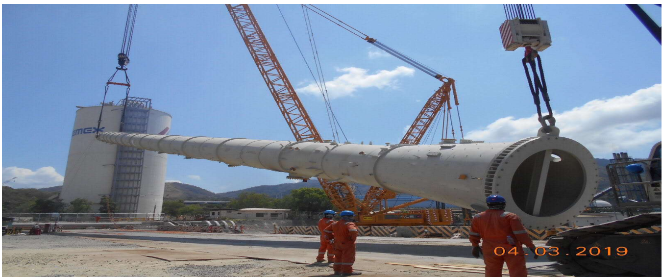
Tandem Lifting of Column weighing 480T and 85 meters high
