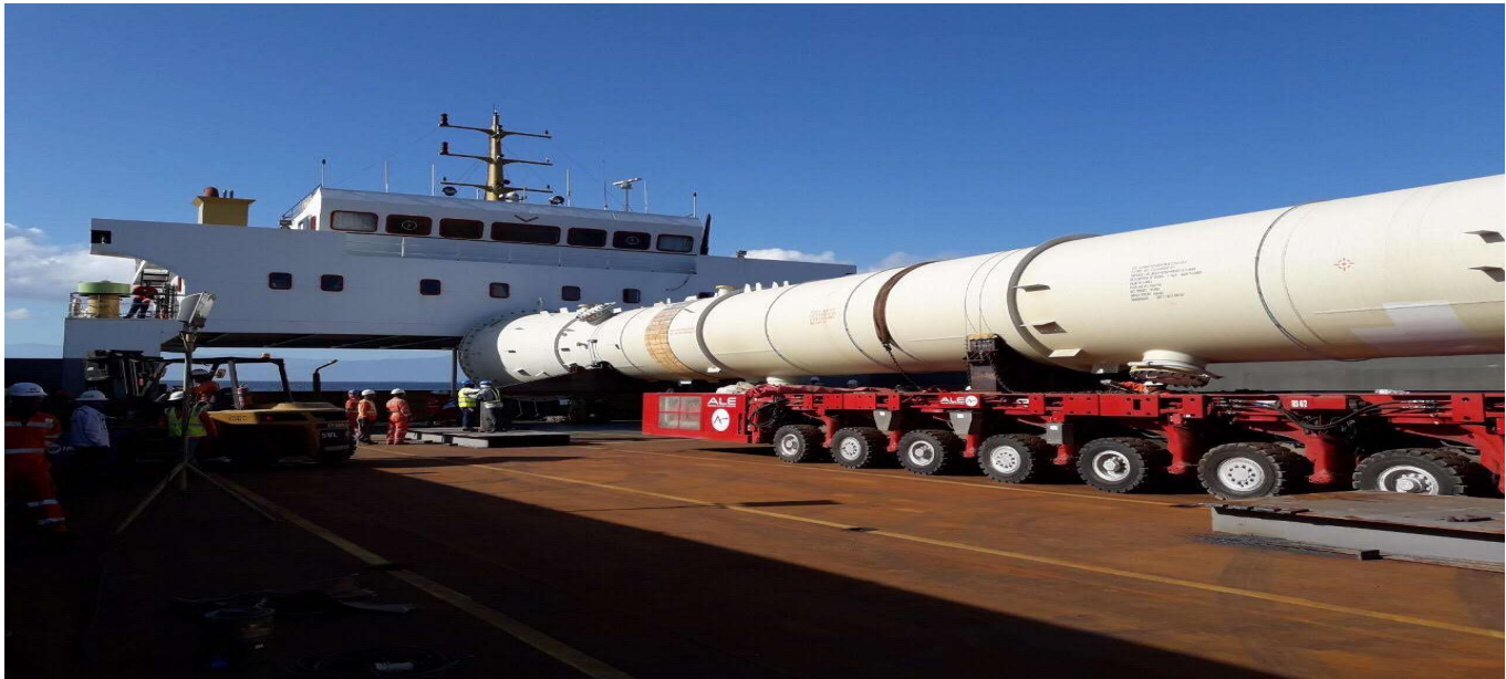
Loading of Column to SPMT
