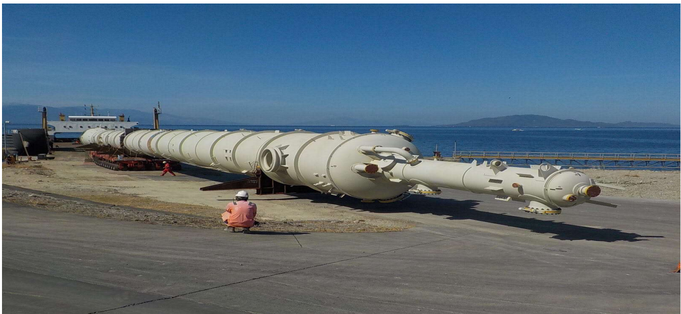
SPMT rolling to Lifting area
