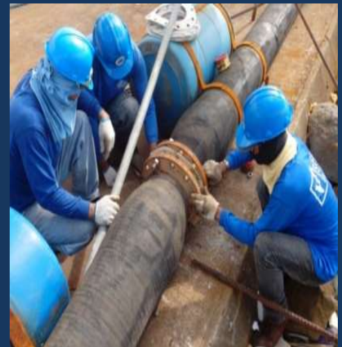
Changing of Marine Hose gasket prior transferring and installation at Jetty Area in preparation for fuel receiving.
