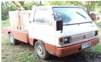
MOBILE GENSET, 10kVA
