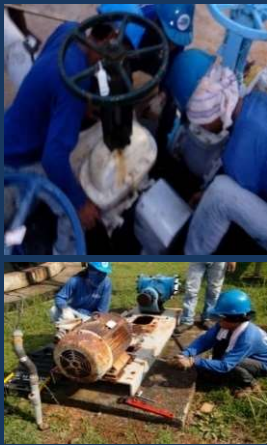
Pump inspection prior pull out for maintenance.
