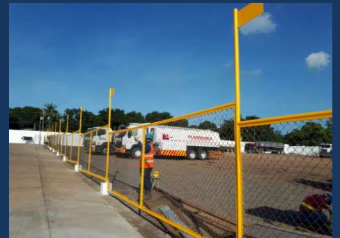
FENCING AT LORRY PARKING AREA
